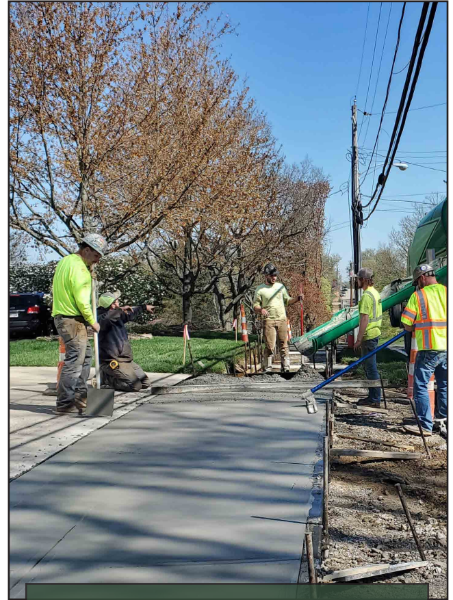
Construction of Sidewalk
